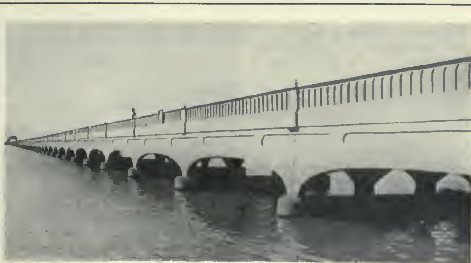
Corpus Christi Causeway—76 - 30 ft. concrete spans with 32 ft. Bascule Bridge.
